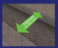
**1.** Ensure max trench width less than 700mm for 44t load. Assess trench stability prior to install.
