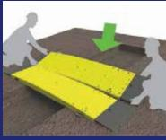
**8.** Lower next plate at an angle so the connectors fit into the slots.
