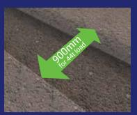
**1.** Ensure max trench width less than 900mm for 44t load, and less than 1200mm for pedestrian load.
