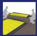
**10.** Repeat previous step until entire trench is covered by inner Road Plate sections.
